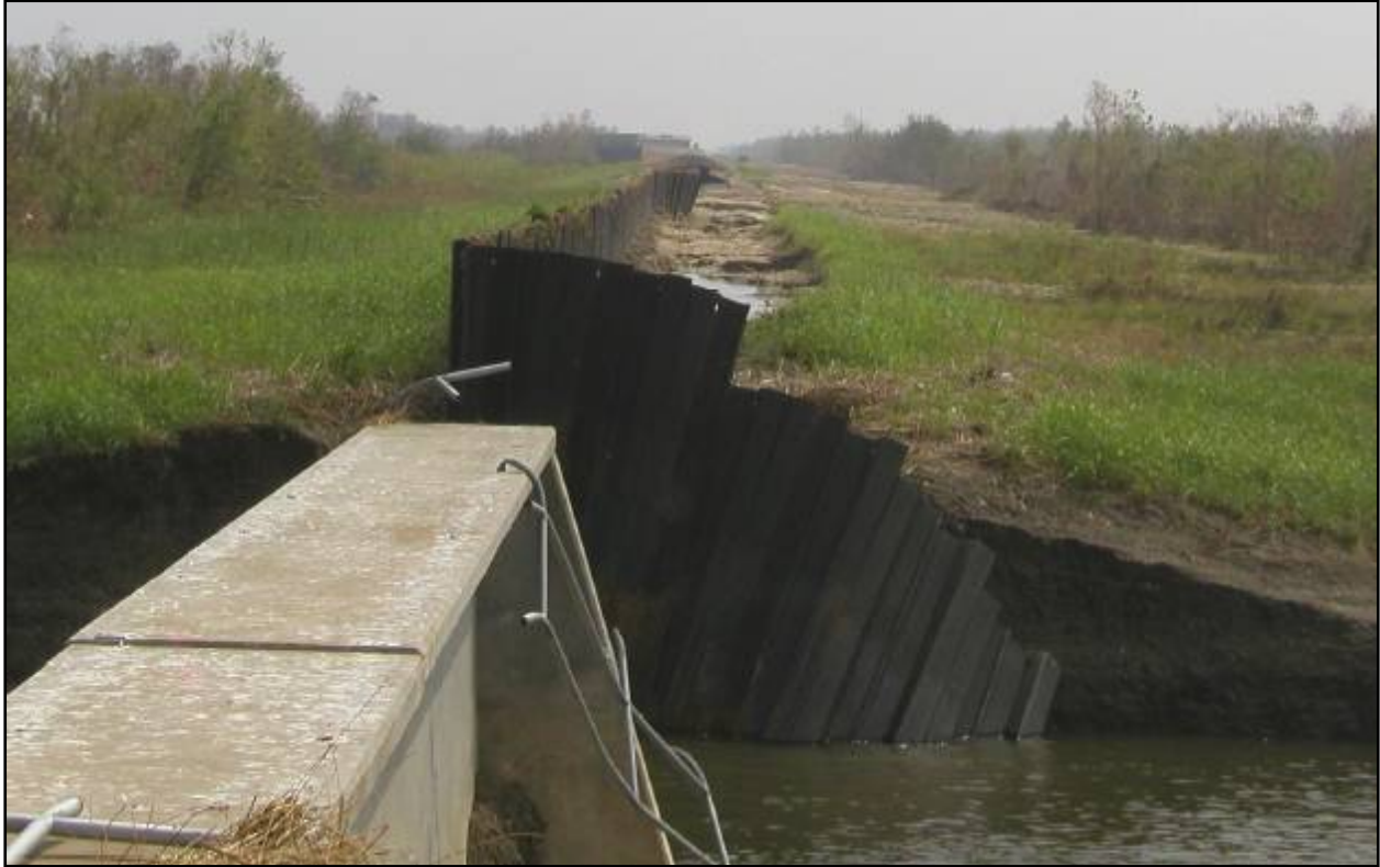
Figure STB 13. Uncapped I-wall Section on Southeast side of Bayou Bienvenue Control Structure (looking southeast along the MRGO)
