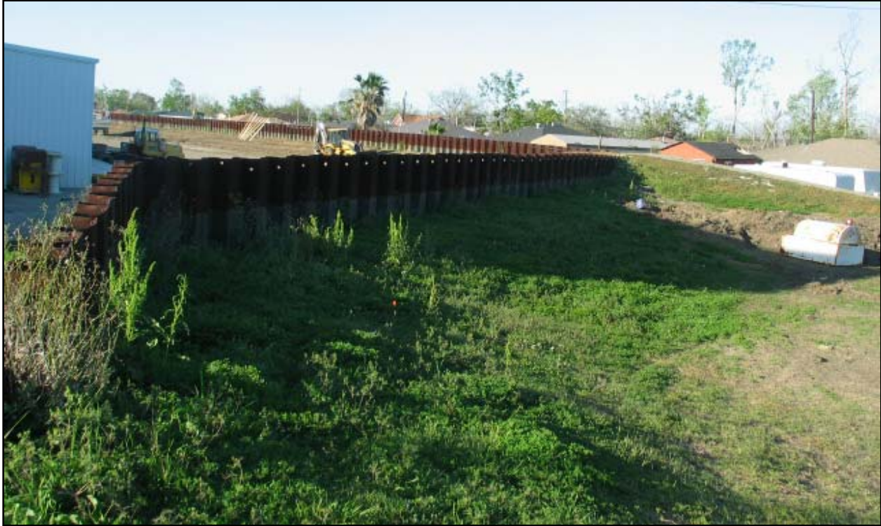
Figure STB 18. Uncapped Sheetpile I-wall near Caernarvon Canal (building on left side is on flood side)
