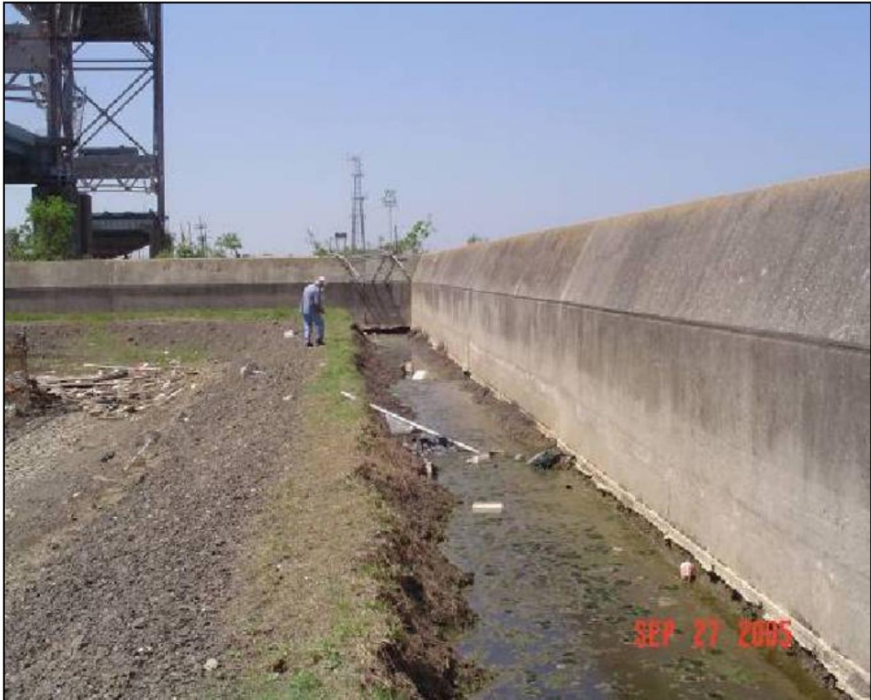
Figure STB 4. Section of Reach STB1 overtopped during Katrina (location is just north of Claiborne Avenue Bridge)
