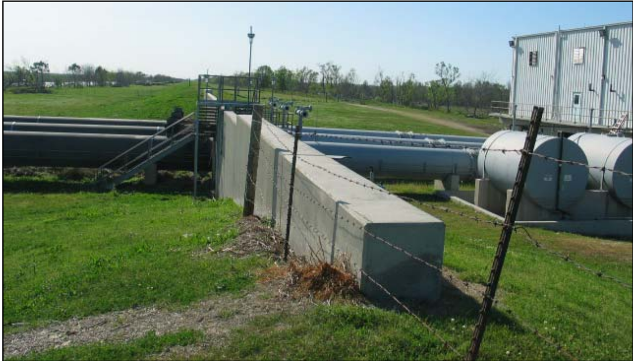
Figure STB 17. Floodwalls surrounding Pump Station #8 pipes (viewed Looking West Along Caernarvon Canal)
