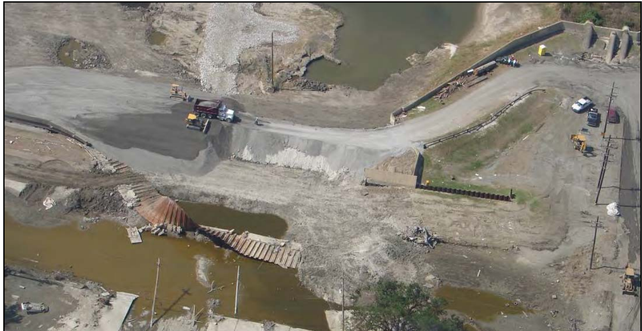
Figure STB 7. North I-wall failure within Lower 9th Ward (Reach STB2) (Note: pipes on right side of photo are associated with Pump Station #5)
