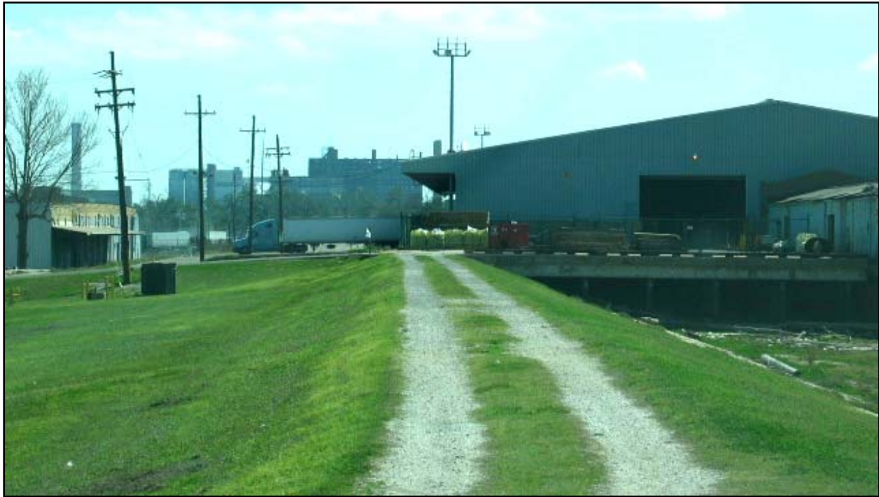
Figure STB 22. End Reach STB31 where levee ties into Dock Facility (Viewed from Reach STB30 side)
