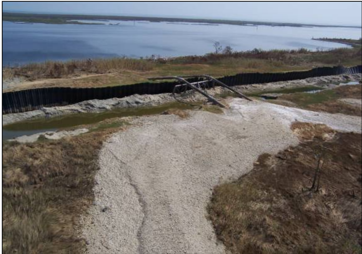
Figure STB 15. Breached I-wall along MRGO
