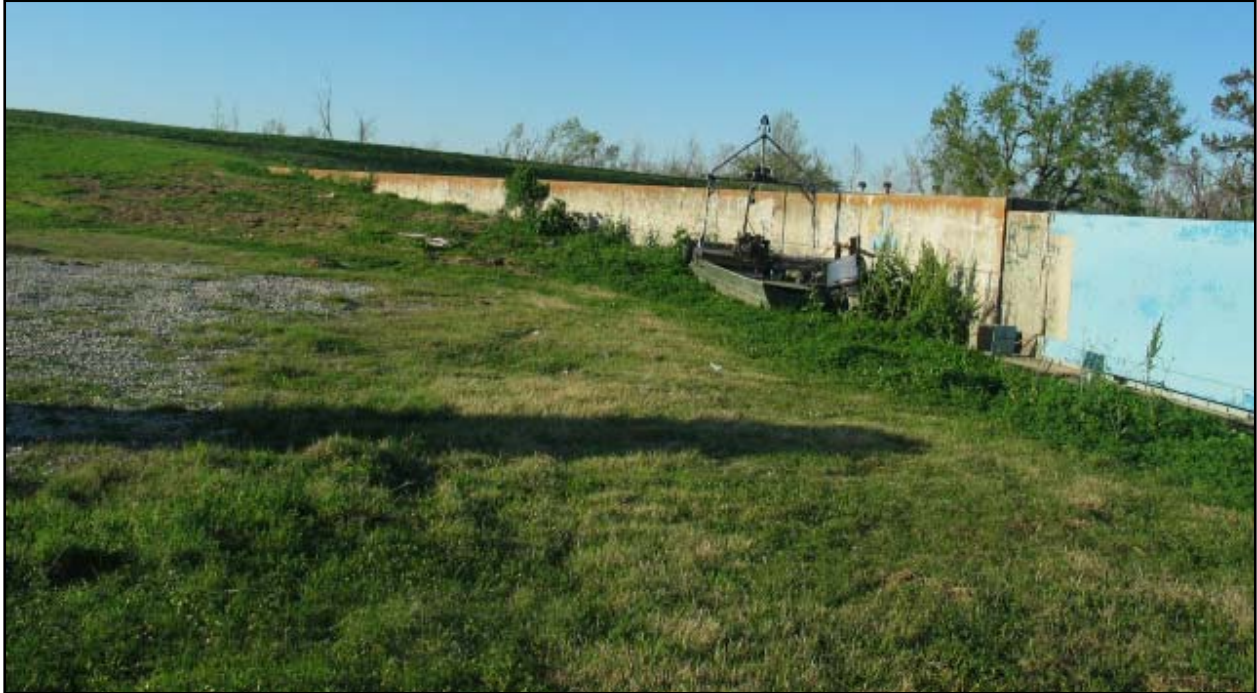
Figure STB 19. Caernarvon Canal Floodwall tie-in to higher MRL (gate is for Highway 39 closure)
