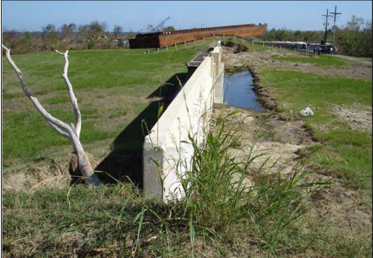
Figure STB 11. Floodwall Northwest of the Bienvenue Structure (Reach STB10) (looking southeast toward Bayou Bienvenue just after Katrina)
