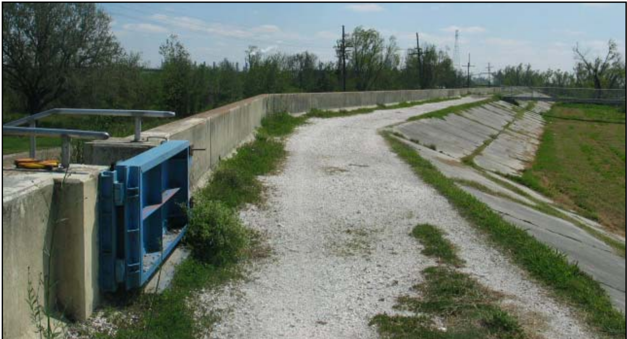
Figure STB 20. Concrete capped I-wall along Miss. River near Battlefield (access closure gate is key point within this reach)
