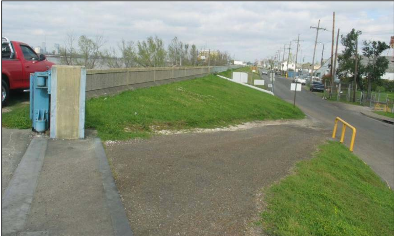
Figure STB 21. Concrete capped I-wall near Domino Sugar Plant (closure represents key point within this reach)
