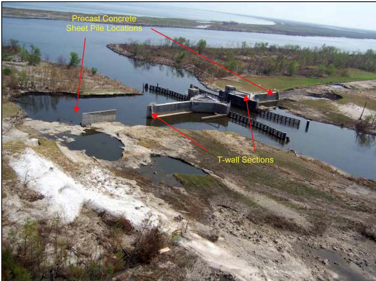
Figure STB 16. Damage at Bayou Dupre Control Structure (note breached section of precast concrete pile wall)
