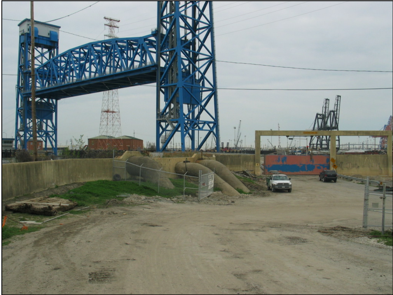
Figure STB 8. Existing T-wall near Florida Ave. Bridge (Reach STB3) (looking from protected side towards IHNC)
